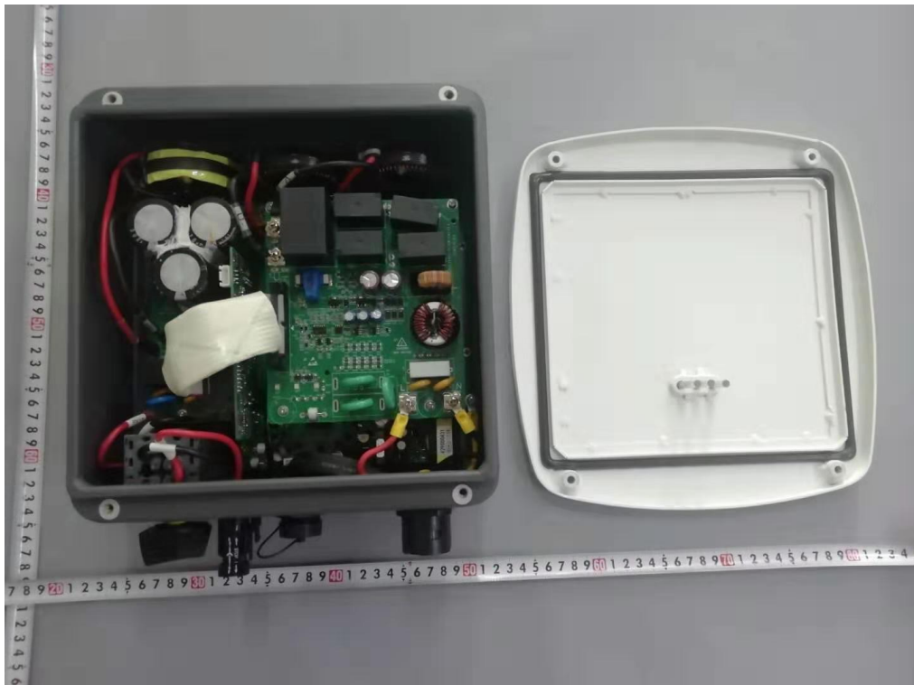
Figura 7. Vista interna Figure 7. Internal view
